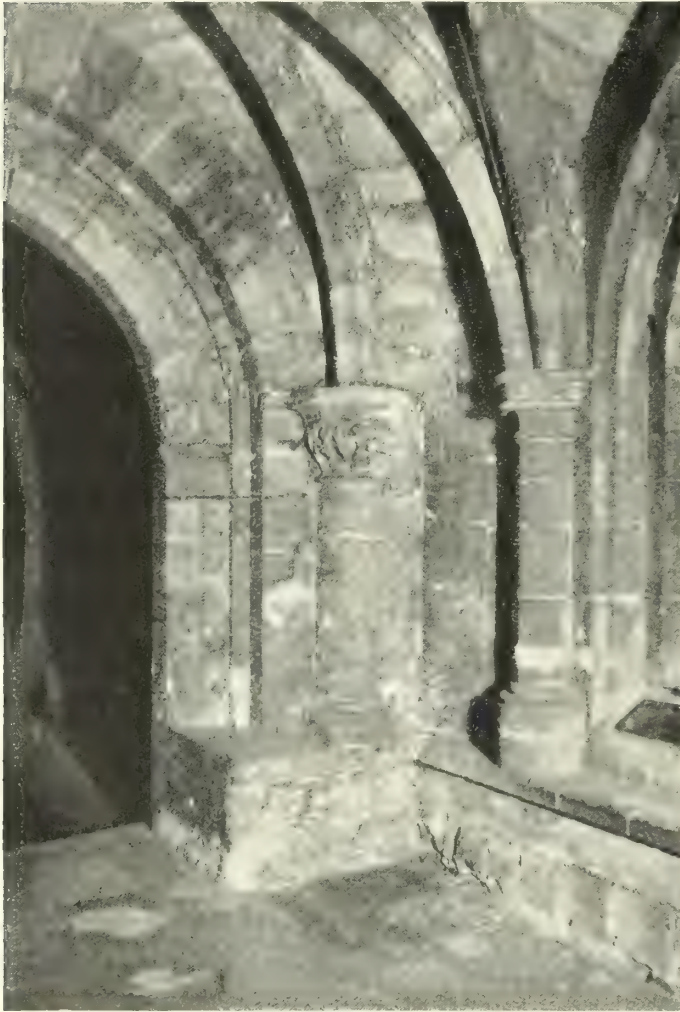
Shafting in South-west corner of Lower Church.
